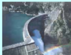
Kurobegawa No. 4 Power Station (Hydropower, 556MW)
