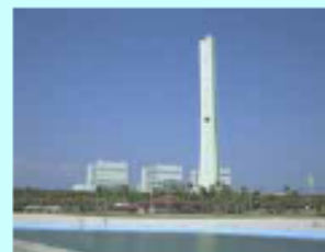
Nankai Power Station (LNG-fired, 1,800MW)
