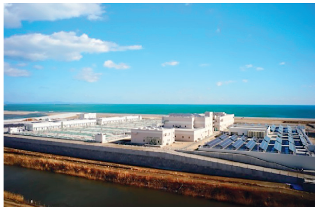
Minami Gamo Wastewater Treatment Plant, where disaster recovery work has been completed
