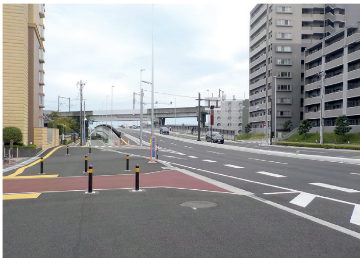
Miyazawa-Nenoshiroishi Road (Minamikajimachi construction area)
