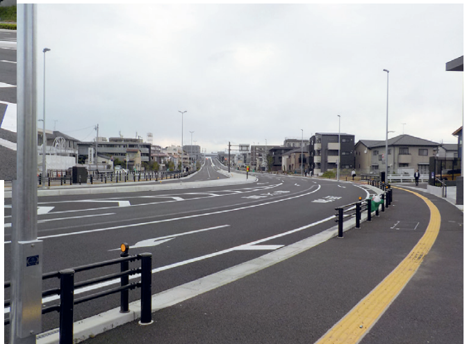
Miyazawa-Nenoshiroishi Road (Funacho construction area)
