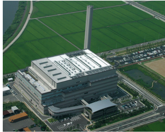
Matsumori Waste Incineration Plant
